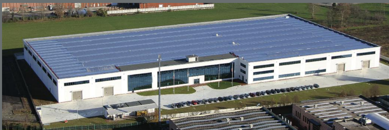
Filtrex Manufacturing Unit #4 - Vignate (Italy)
