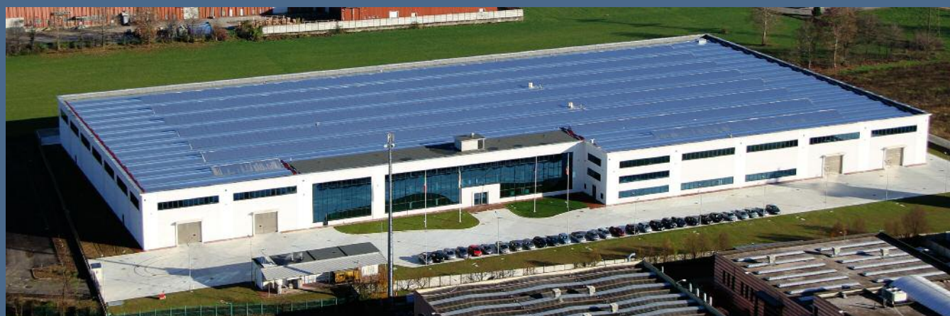
Filtrex Manufacturing Unit #4 - 22,000 covered sqmt - Vignate (Italy)
