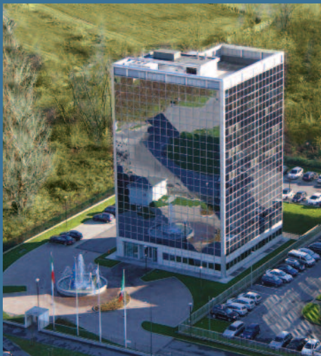
Filtrex Corporate Headquarters - Milano (Italy)
