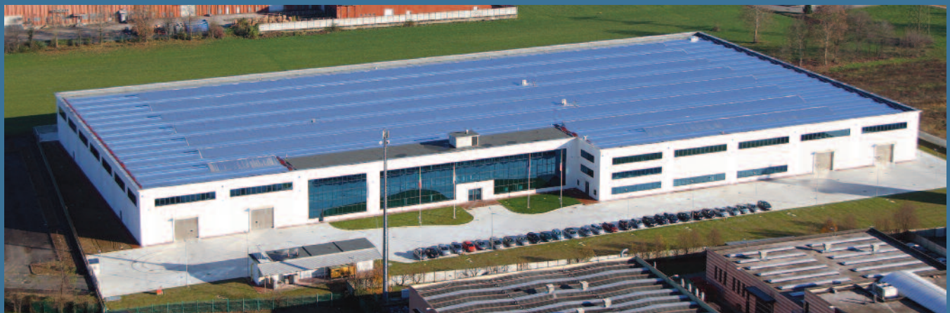
Filtrex Manufacturing Unit #4 - 22,000 covered sqmt - Vignate (Italy)
